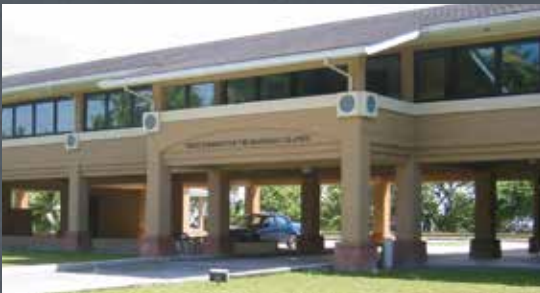
The Trust Company of the Marshall Islands, Inc. located in Majuro, capital of the RMI.
